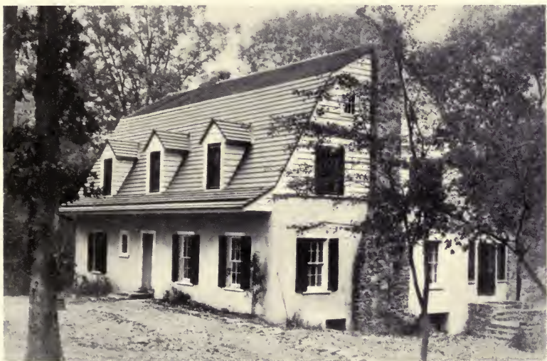
FIGURE 2. Rammed earth house. Residence of Dr. H. B. Humphrey, Cabin John, Maryland. This house, of Dutch Colonial design, was erected on a foundation of poured-concrete blocks.
